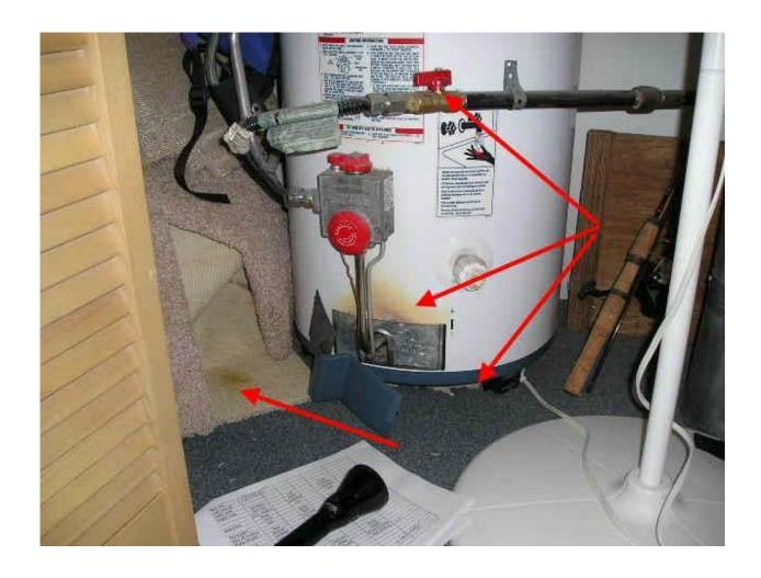
The water heater and furnace were in the same closet. The louver doors did not allow for enough combustion air. This is the cause of the brown heat marks on the water heater. The owners also had carpet and Christmas wrapping paper stored in the same closet. Notice the char mark on the carpet. They are very lucky a fire did not occur.
