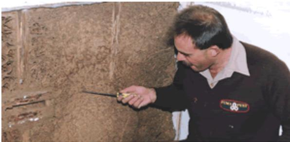
The picture on the left shows a termite inspector examining an above ground termite subsidiary nest built inside a wall cavity of a home.
